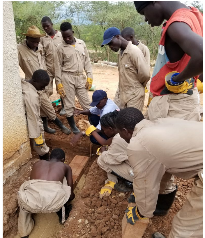
Community Scouts build a new ranger station Murchison Falls National Park - Uganda
